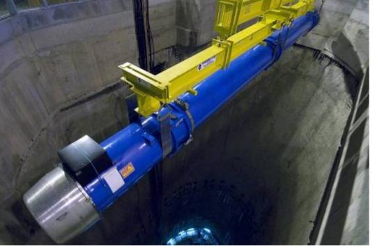
Only one access point for 15 m long dipoles, 35 tons each
