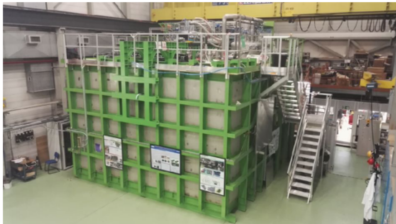
Nov 2016 : control racks, DAQ and cryogenics installed, cabled and tested
