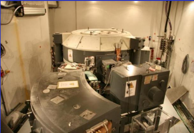
Cyclotron S2C2 (CAL)
