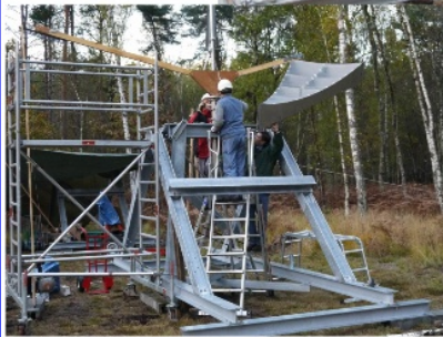
truck part of the dish.
