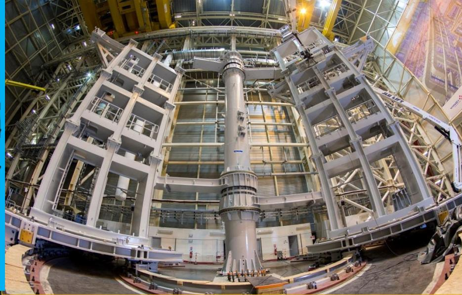
Before being integrated in the machine, the components are pre-assembled in this 6,000 m<sup>2</sup>, 60-metre high building. The Assembly Hall is equipped with a double overhead travelling crane with a total lifting capacity of 1,500 tons. Load tests, both static and dynamic (1,875 – 1,650 tons), were finalized in December 2017. To the right, the installation of the giant tool (SSAT-1) is ready for making the 1<sup>st</sup> sub-assembly of a 1/9 module
