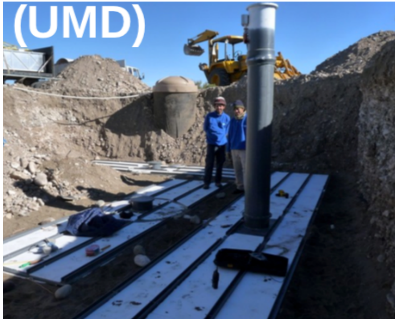
Underground muon detectors (2.3 m soil for shielding)
